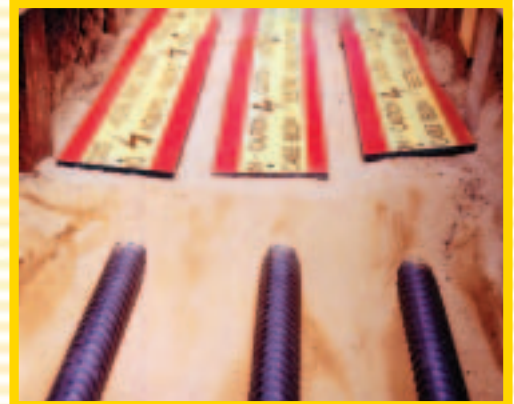
STOKBORD® is the modern, safe solution to underground services protection.
