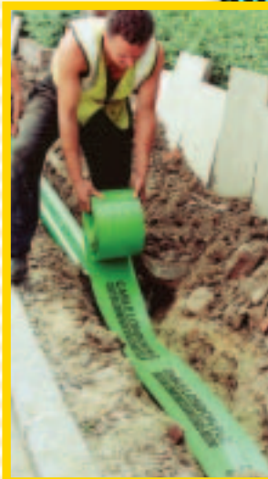
Communications cable protection roll
