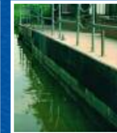
Stokbord used for lining a canal jetty
