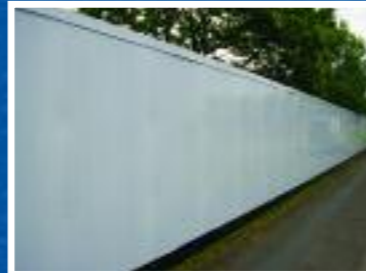
Hoardings made from recycled HDPE
