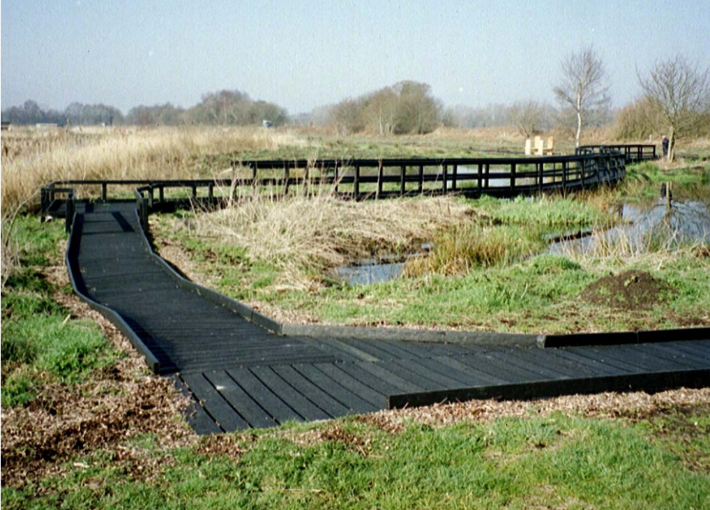
Raised boardwalk with woodchip fringe, Ham Wall Reserve
