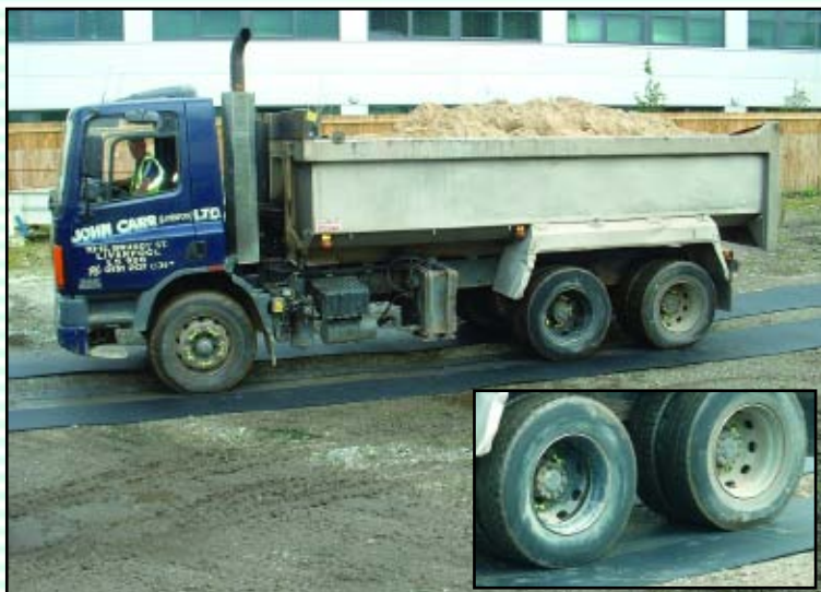
STOKMAT® used as ground protection on building sites
