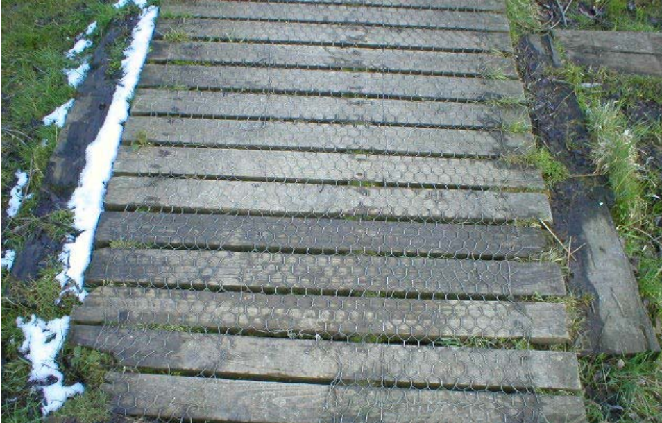
Howden Marsh – wooden boardwalk with wire mesh
