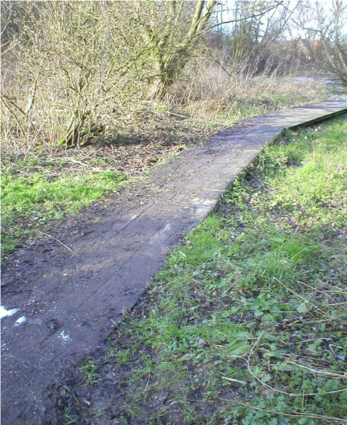
Howden Marsh – railway sleepers boardwalk with wire mesh
